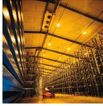
The specific VESDA products installed are LaserPLUS detectors. These offer a simple, cost-effective solution for the protection of temperature controlled facilities. "Our consultants explained that most fire protection technologies which are designed to operate in freezing conditions are not capable of early warning detection and are prone to being damaged by production equipment", commented Wayne Aspeling, General Manager: Gauteng Manufacturing.
